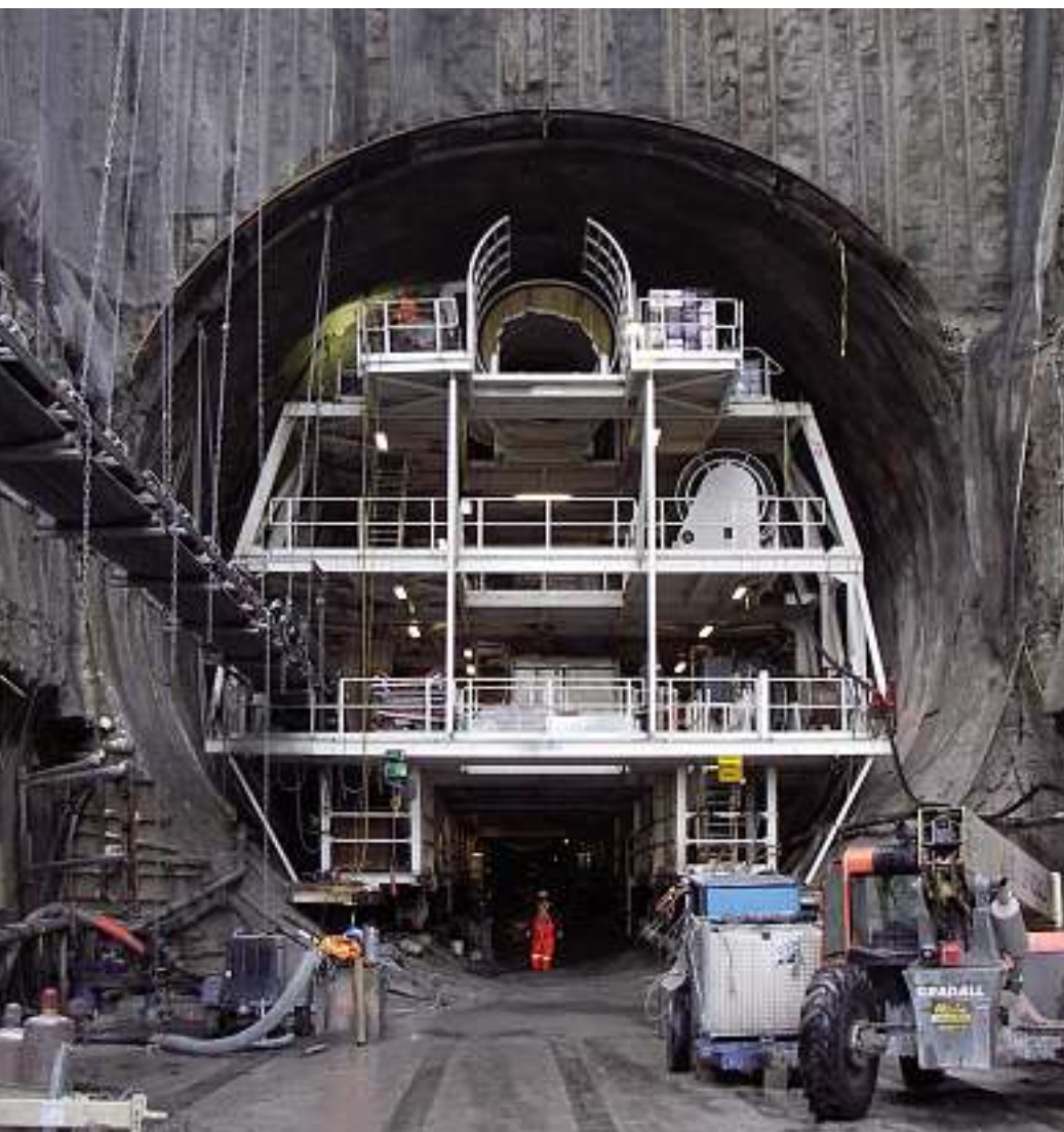
World's largest open hard rock tunnel boring machine, Niagara Tunnel, Canada
