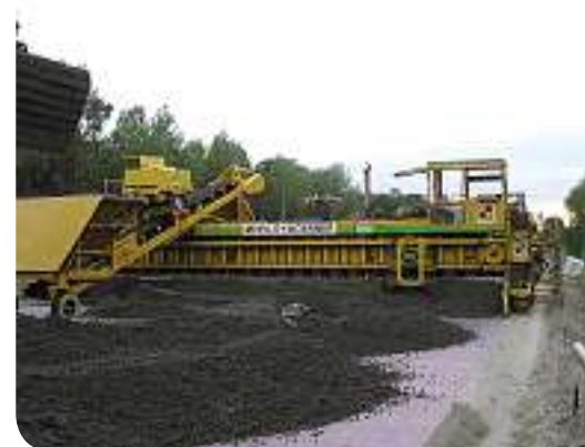
GSF19 concrete finishing machine in action
