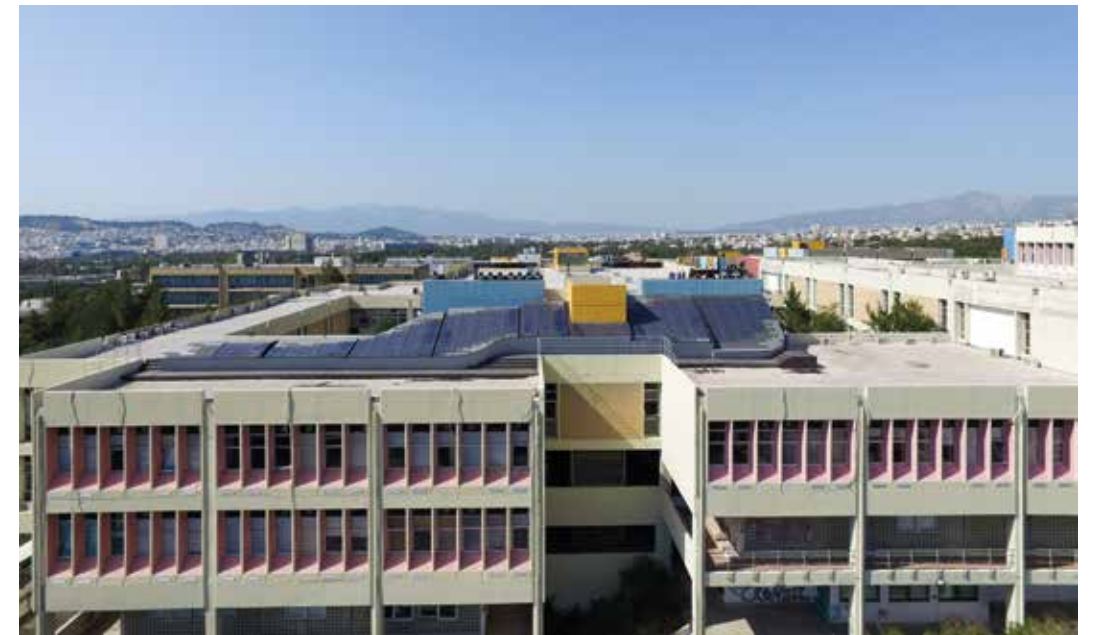
◀ Photovoltaikfassade am Z3 in Stuttgart / Photovoltaic facade on the Z3 building in Stuttgart
